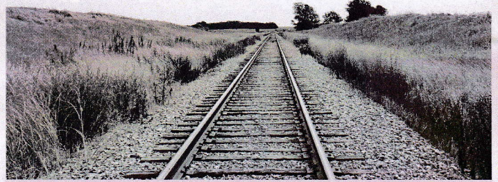
This modern photo of a railroad cut was taken about two miles to the east of the Tracy Cut, which was a protagonist in The Long Winter . During the Hard Winter, the cuts were much narrower, which is what caused snow to become trapped. In the years after the winter, cuts were widened to prevent that problem. Photo by author.
