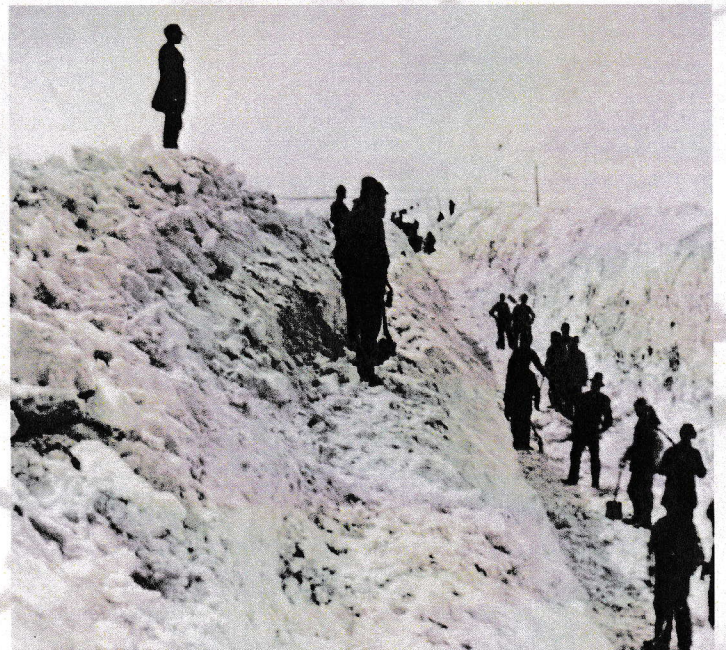
Elmer & Tenney photo taken late in the winter, this one showing the tiers so that the snow could be tossed away from the tracks. Photo courtesy Chicago & North Western Historical Society
