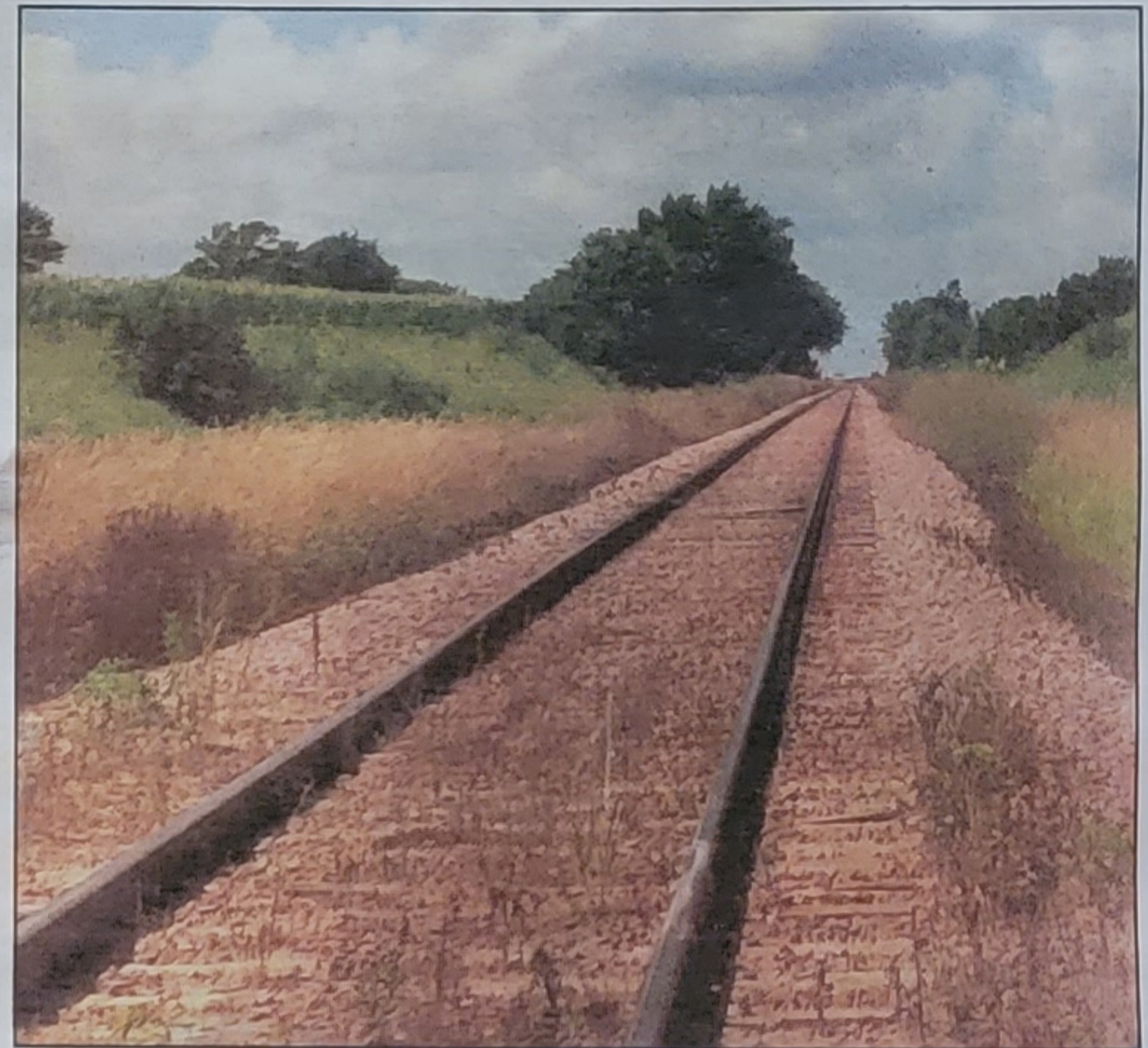
THE "TRACY CUT" is still visible today, 4.5 miles west of Tracy, although wider and less steep than it was during the winter of 1880-81. Photo / Marcy Schramm.
