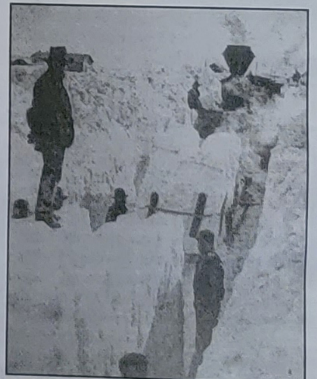
CREWS OF SHOVEL-WIELDING MEN were often overmatched by Mother Nature, in trying to keep tracks clear of snow during the arduous winter of 1880-81. This Chicago & Northwestern Historical Society photo, which is displayed at the Wheels Across the Prairie Museum, shows men attempting to clear passage for a train near Sleepy Eye in April of 1881. Similar epic snow-clearing efforts were also often needed in a snow-clogged cut west of Tracy.
